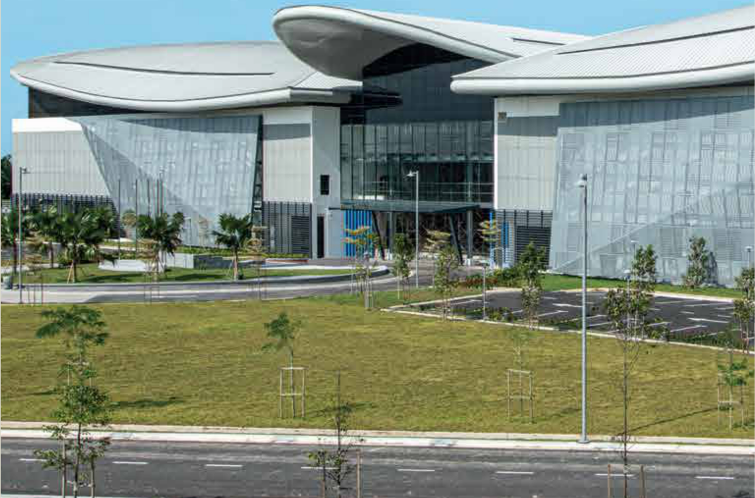
Kuala Lumpur Air Traffic Control Complex
